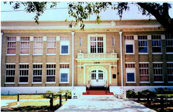
Graham Elementary Renovations TAMPA
